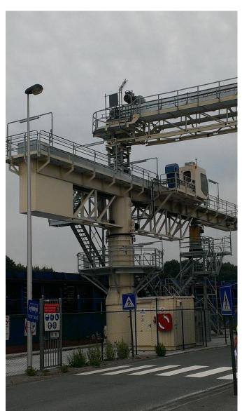
In 2015, a loading crane was treated with a duplex system: a ZINGA base coat and a PU sealing coat. This application was handled by Buijsseon a blasted surface.
