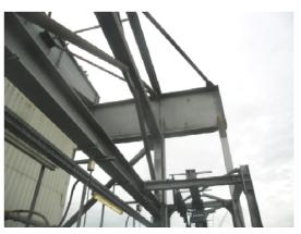
The beams were treated with 2 x 60  $\mu$ m DFT after steel fabrication at Victor Buyck to provide a good corrosion protection in a harsh industrial environment.
