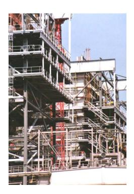
For the expansion plans in 1997, ZINGA was prescribed for corrosion protection of 7500 m<sup>2</sup> construction steel by the engineering company Tractebel.
