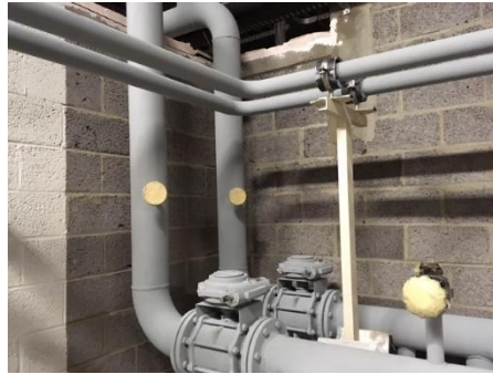
After repairs with ZINGA
