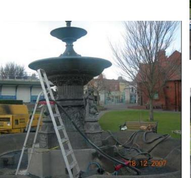
Blast cleaning to remove the old paint. (picture taken on 18-12-2007)
