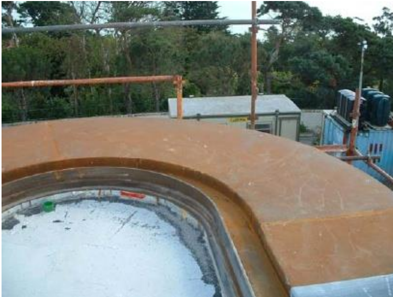
Left : View of canopy corner from above, showing guttering.
