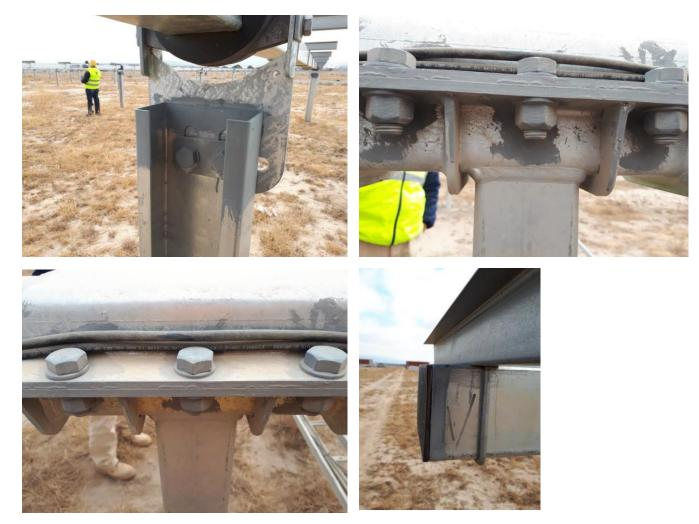
System: Manual surface preparation ZINGA by brush: 60-80 μm DFT
