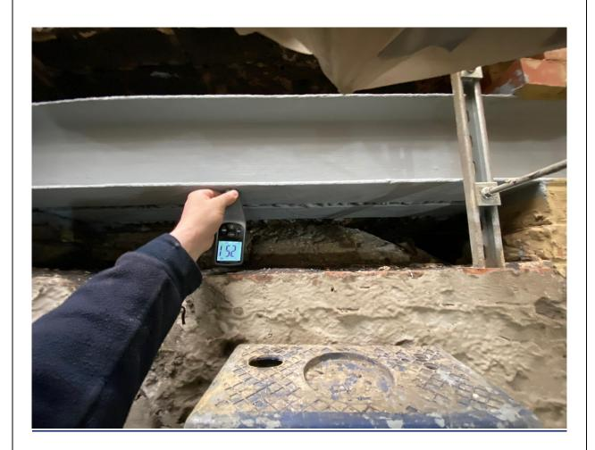
8. This reading was taken over an old beam, so surface corrosion defects could account for this high reading.
