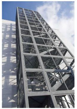
The fire escape was originally hot-dipped and was reloaded with ZINGA to give it renewed galvanic corrosion protection.
