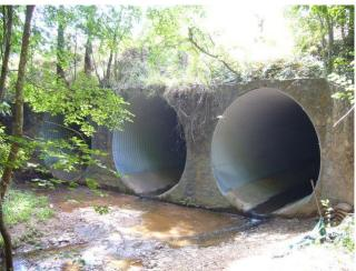
The below pictures reveal the general conditions of the culverts. This is quite common in most states of Australia. As bad as the corrosion looks, in most cases it did not penetrate through the existing galvanized steelwork.
