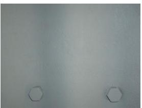
All edges, bolts and nuts have been stripe coated before the application of the full coating system to ensure a perfect seal and total protection.
