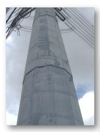
These pictures were taken in 2003, 4 years after the application of ZINGA on old, damaged hot-dip and no rust was detected at all.
