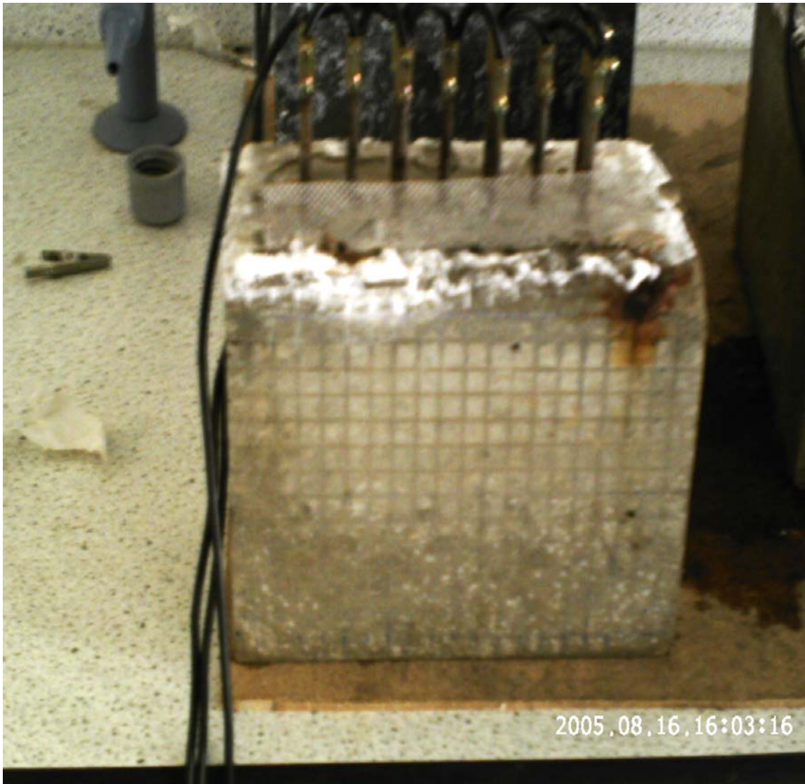
Concrete block three (impressed current) after the experiments.
