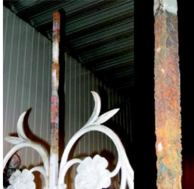
Composition highly attacked by corrosion
