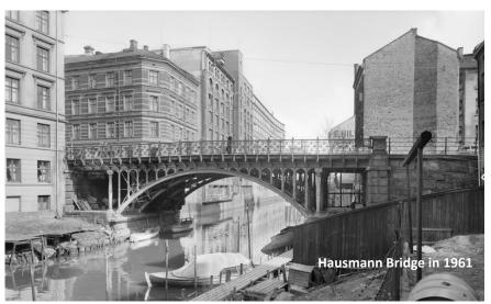
The bridge was built in 1892 by the Christiania Municipal Road Administration, in cast iron with detailed decorations. The bridge was rebuilt (extended double-wide) in 1982. The new bridge was completed in similar style as the original, including copies of original details in cast iron construction and the old railing was retained.
