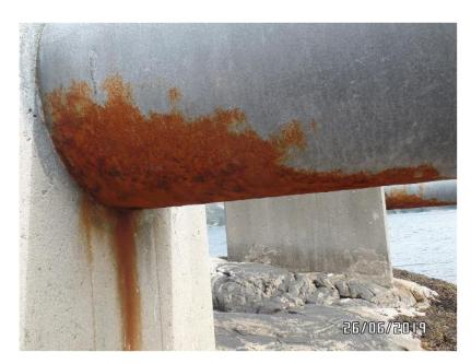
This project shows clearly that when preparation and /or application is not done up to the best standard on the whole structure and under such harsh conditions, failures can occur.
