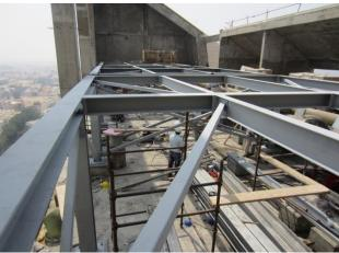
During construction of the building from 2010 until 2013, **ZINGA** was specified instead of hot dip galvanization (by **Saudi Diyar Consultant**) for about 30 tons steel beams at the water treatment station located at an open area on the 16th floor of the Eastern tower.
