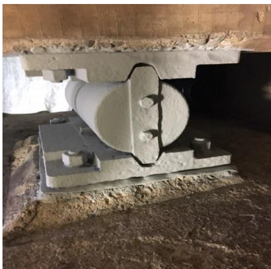
After application of ZINGA . The picture on the right shows shiny metallic zinc after a coin rub test was performed.
